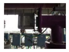
The SafEye Duct Mounted Gas Detector uses its source and detector to detect gases at the 3.4m wavelength with the ability to determine the concentration of the gases, before they reach explosive levels. Relevant precautions can then be taken to ensure that an explosion doesn't occur.
