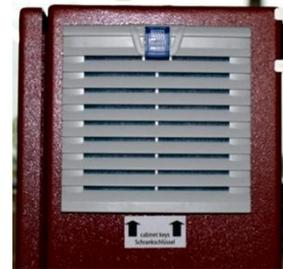
Replace the exhausted filter mat through a new one.
