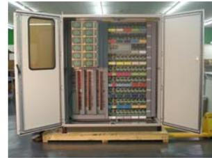
In order to tie the new sensors into the existing deluge system, GDS Corp and the customer co-designed a custom cabinet with twelve C1 *Protector* controllers, sensor input boards, channel relay output boards and interposing relays that eventually controlled the field-mounted deluge valves. As a result of the modular design of the C1, the input modules, output modules and display could be mounted separately, simplifying wiring and construction.
